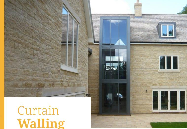
Our lightweight aluminium curtain walling systems are engineered to offer high performance solutions for new and refurbished buildings.
